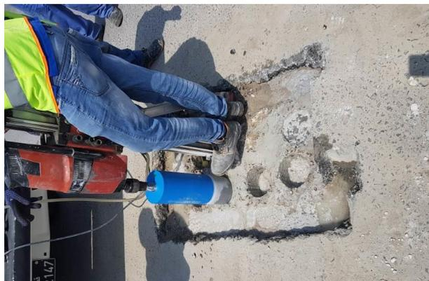
**Fig. 5 Self-hardened RCA subbase exposed after 4 years in service during coring.**
