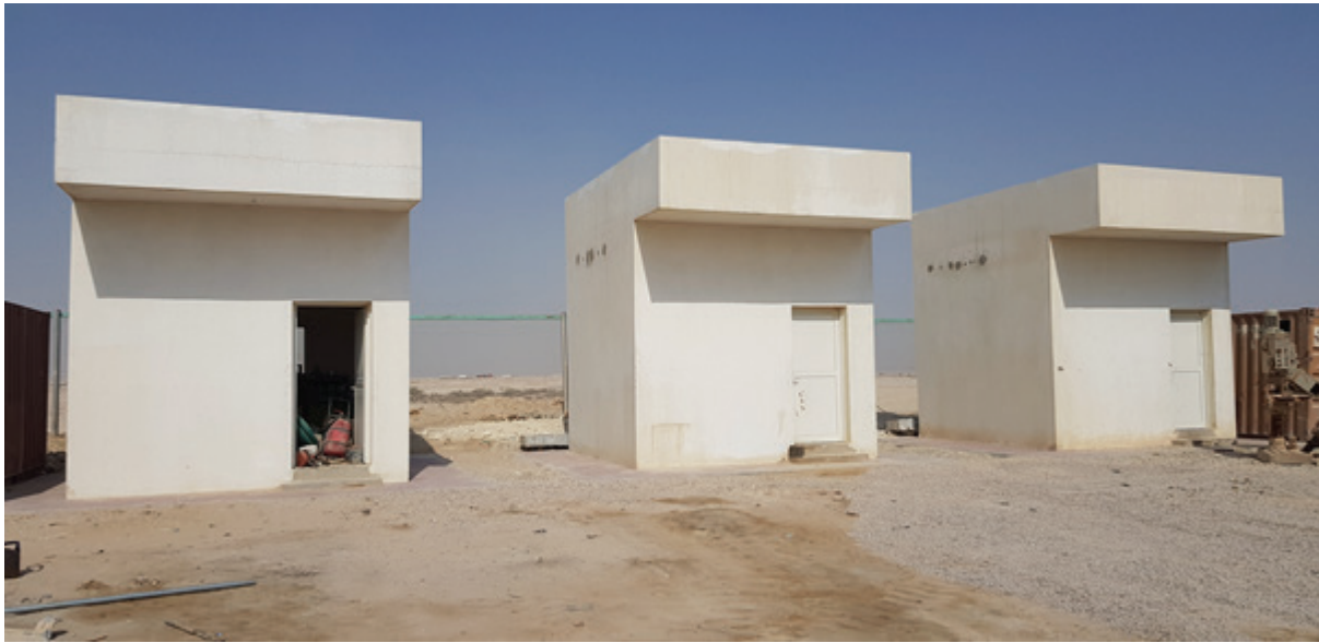
Figure 5-16 Trial buildings, 4 years after construction: control (100%) gabbro on left; 50% Wadi gravel in centre; 100% Wadi gravel on right.
