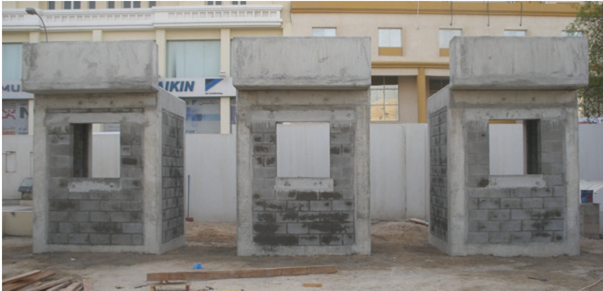
Figure 5-1 EW and CRF building trials immediately after construction
