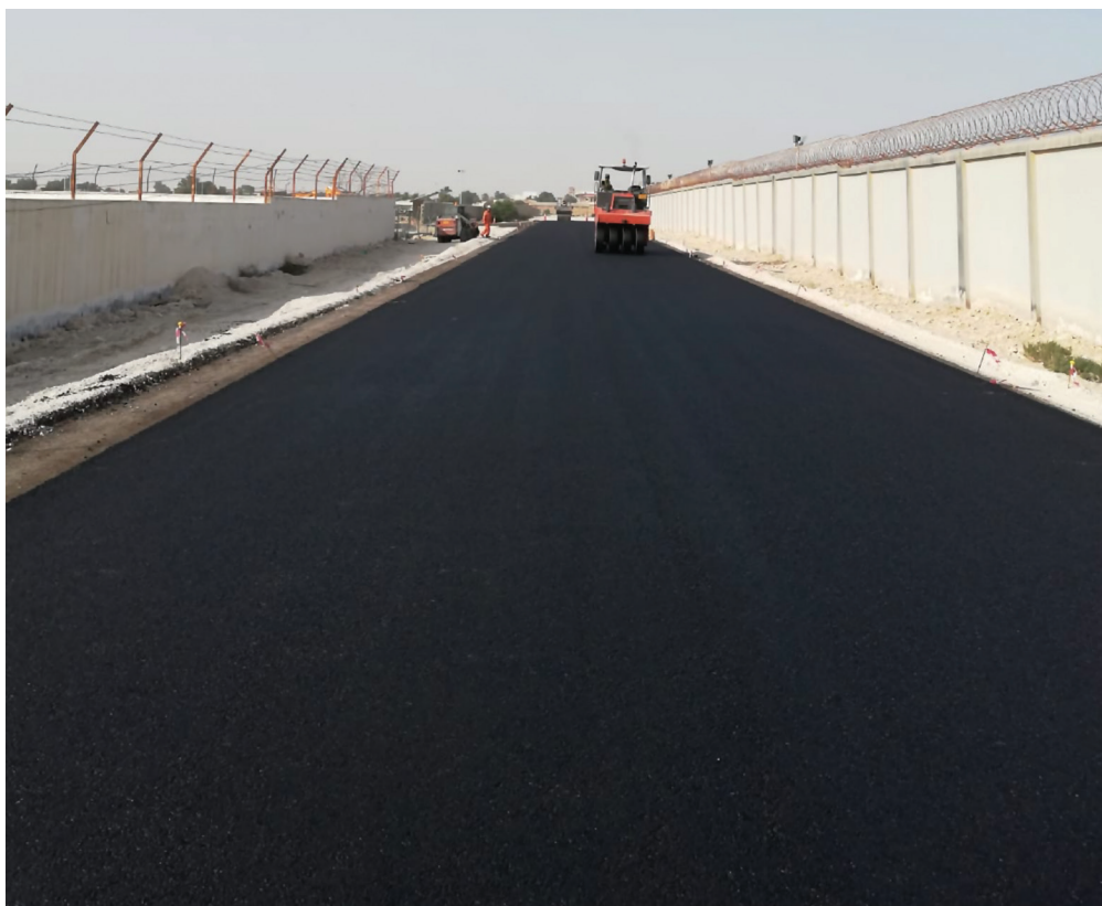
Figure 4-14 Construction of CRMB road section – Al-Bustan Street
