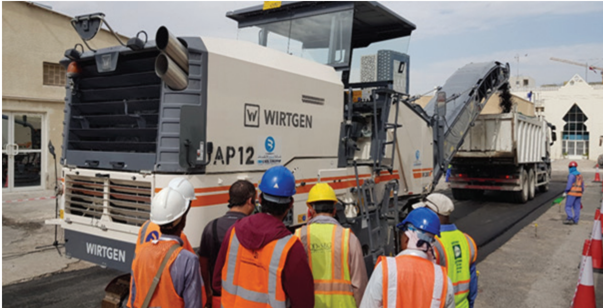
Figure 3-5 Ashghal demonstration on asphalt milling to their contractors
