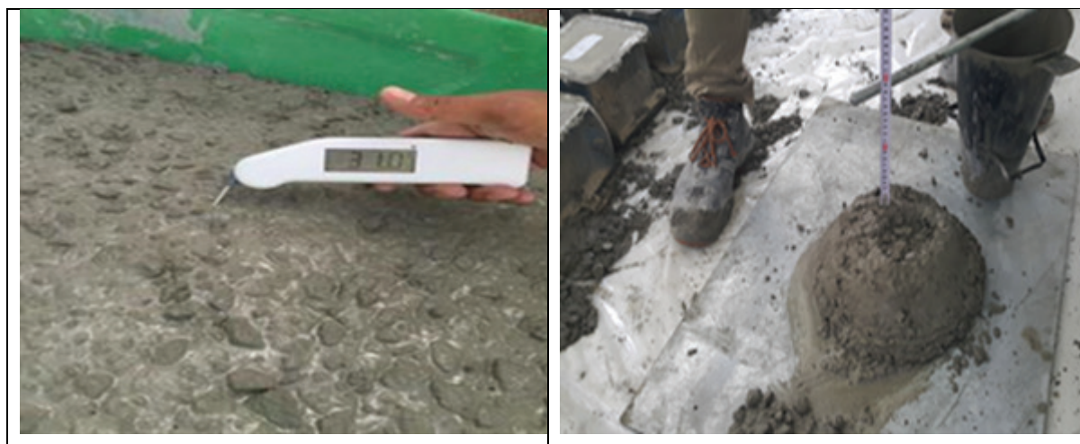
Figure 5-12 Measurements of concrete temperature (left) and slump (right) on site
