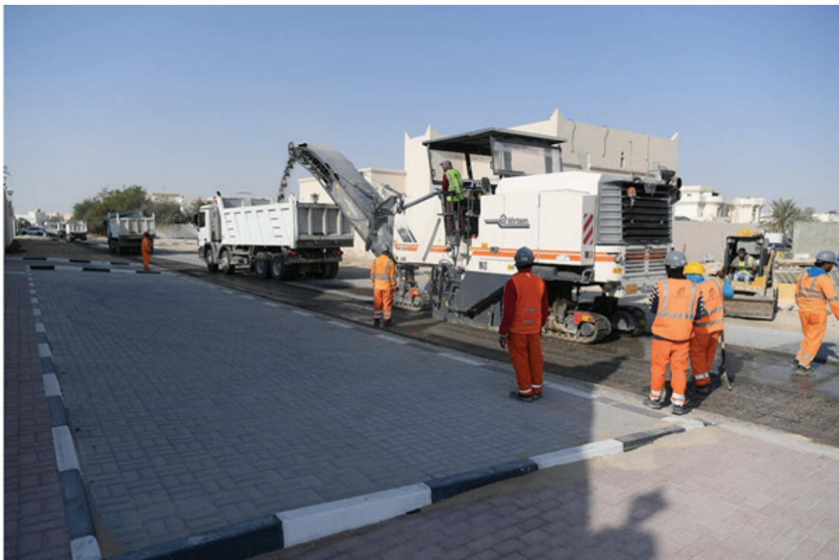
Figure 4-5 Milling of old asphalt road – Izghawa project
