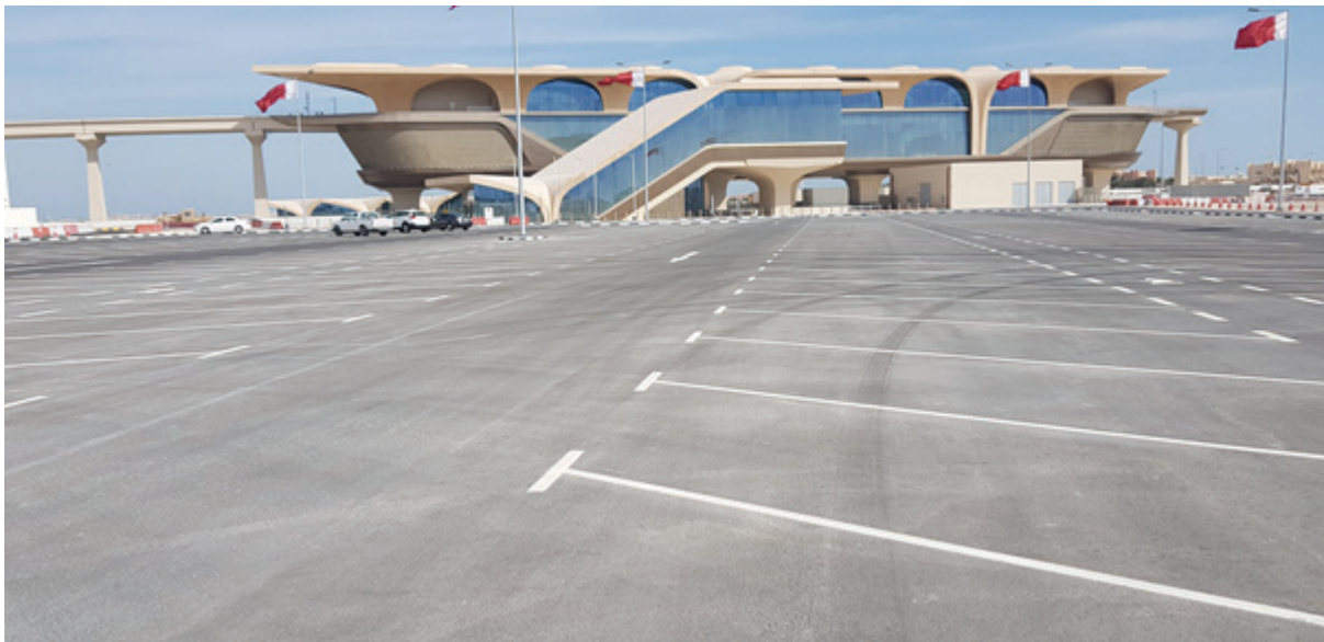
Figure 4-1 Al-Wakrah Metro car park – RAP asphalt
