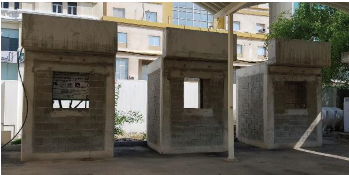
Figure 5-2 EW and CRF building trials after 5 years in service
