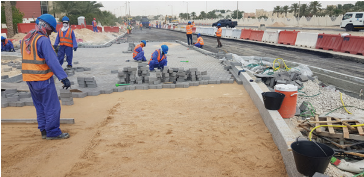
Figure 6-11 CBM 3 overlaid with sand and paving blocks – Katara Metro Station
