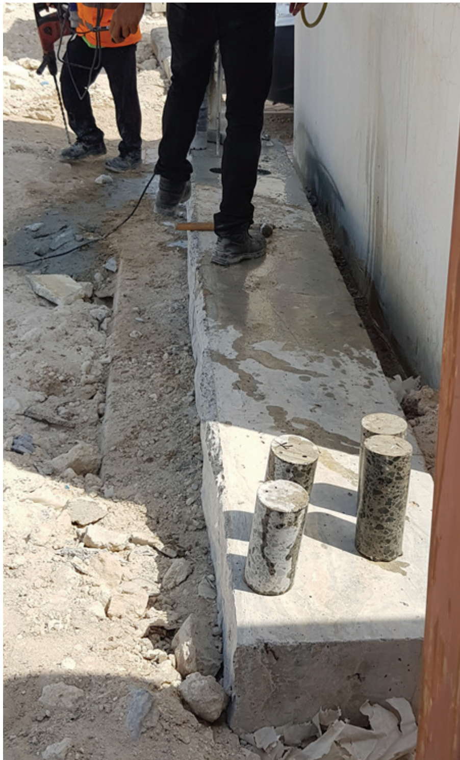
Figure 5-11 Additional beam cast for coring and long-term monitoring behind buildings.
